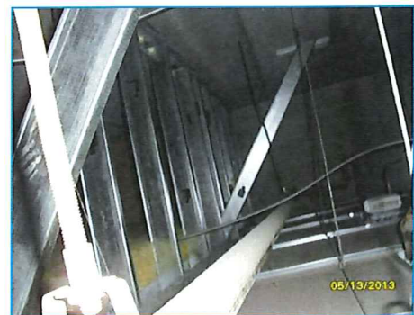
Soffit at Prison with no air barrier
