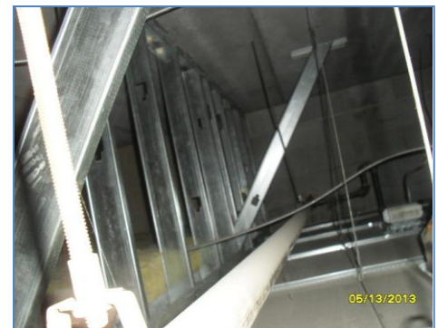
Soffit at Prison with no air barrier
