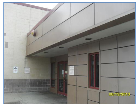
Soffit at Prison with no air barrier
