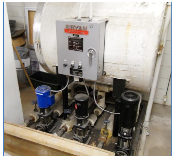
Typical Bryan Water Tube Steam Boiler
