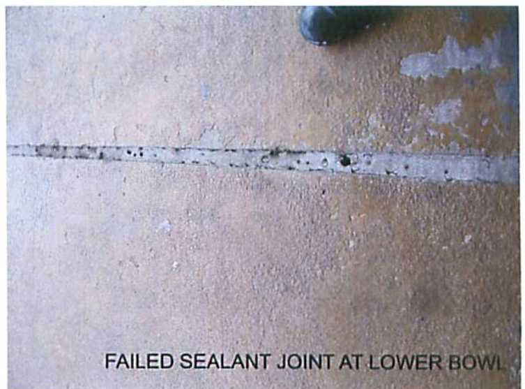
FAILED JOINT SEALANT / SPALLED CONCRETE NOSING AT LOWER BOWL AISLE
