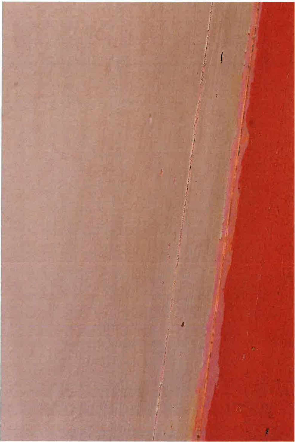
scratch in ochre paint reveals faded red under
