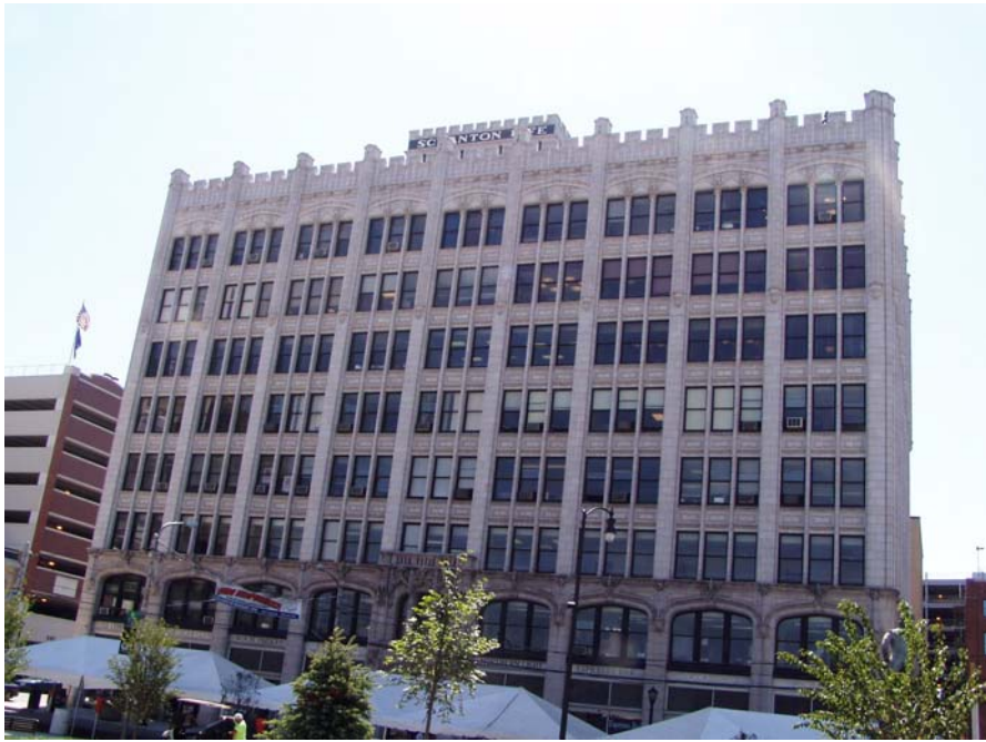
View of building looking across Spruce Street
