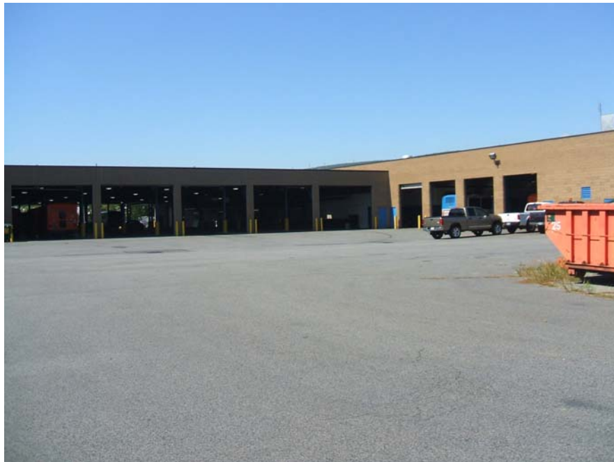
View of garage and repair bays
