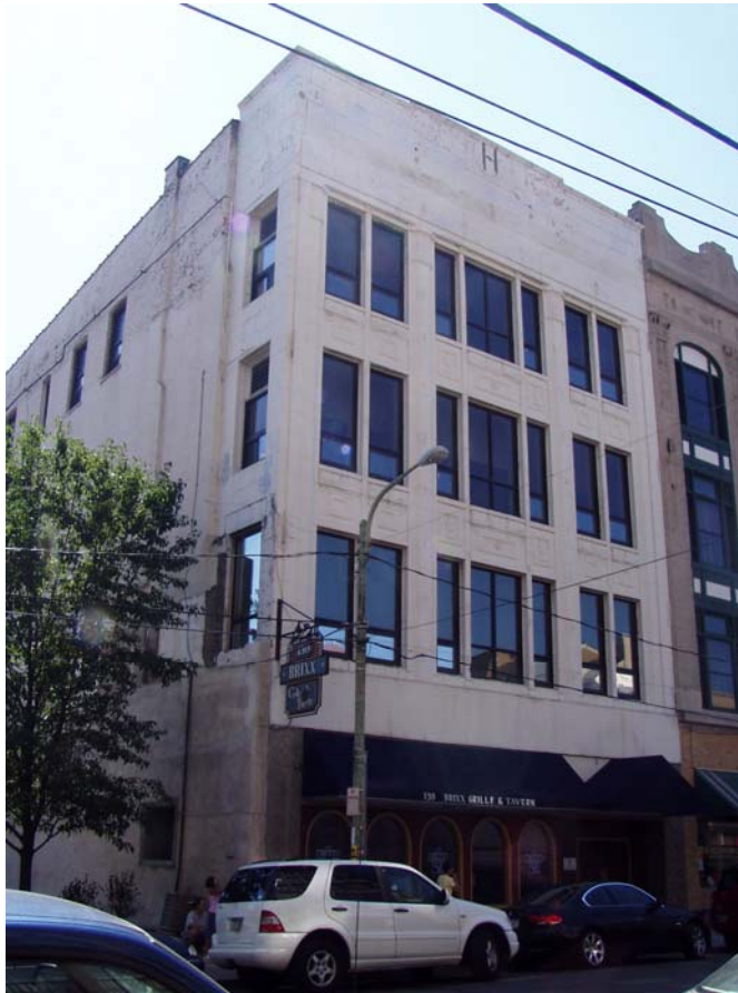
View of building from North Washington Avenue
