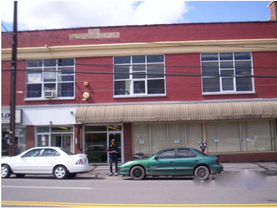
View of front of building from Wyoming Ave.
