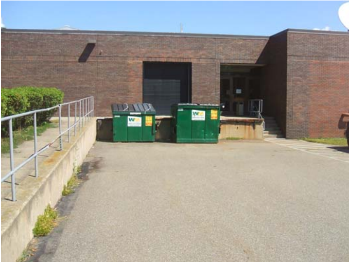
Looking north showing loading dock
