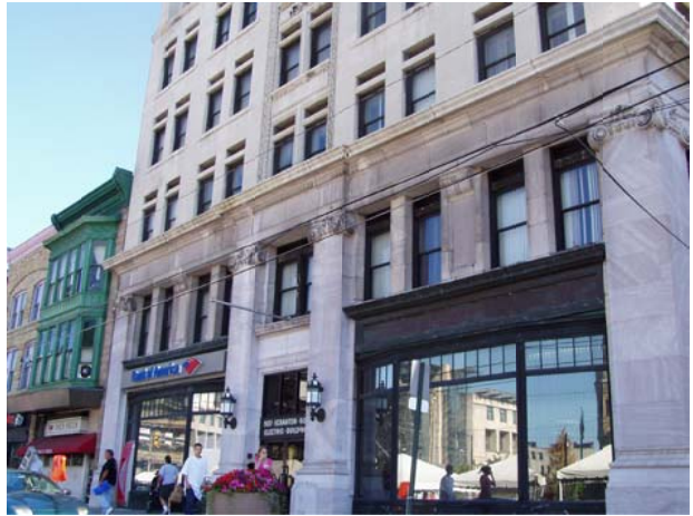
SCRANTON ELECTRIC BUILDING
