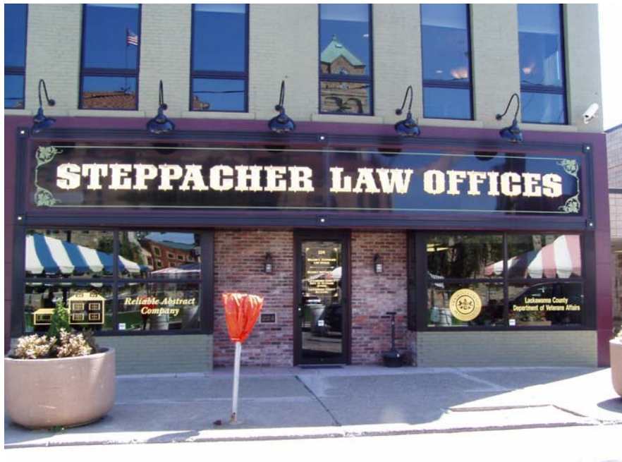
View looking across Adams Avenue showing county offices on right
