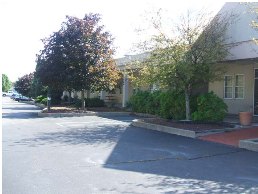
View of building looking northeast
