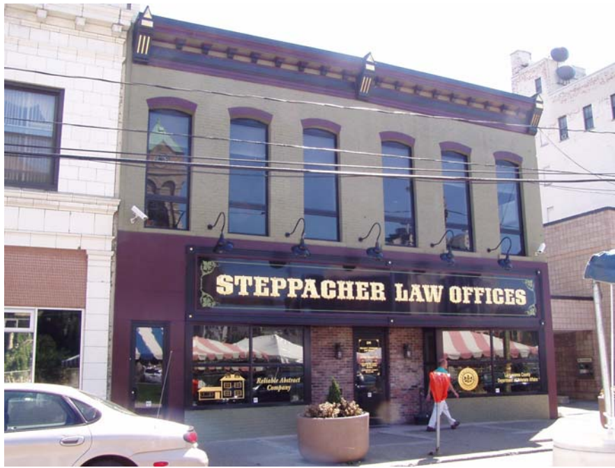
View looking across Adams Avenue
