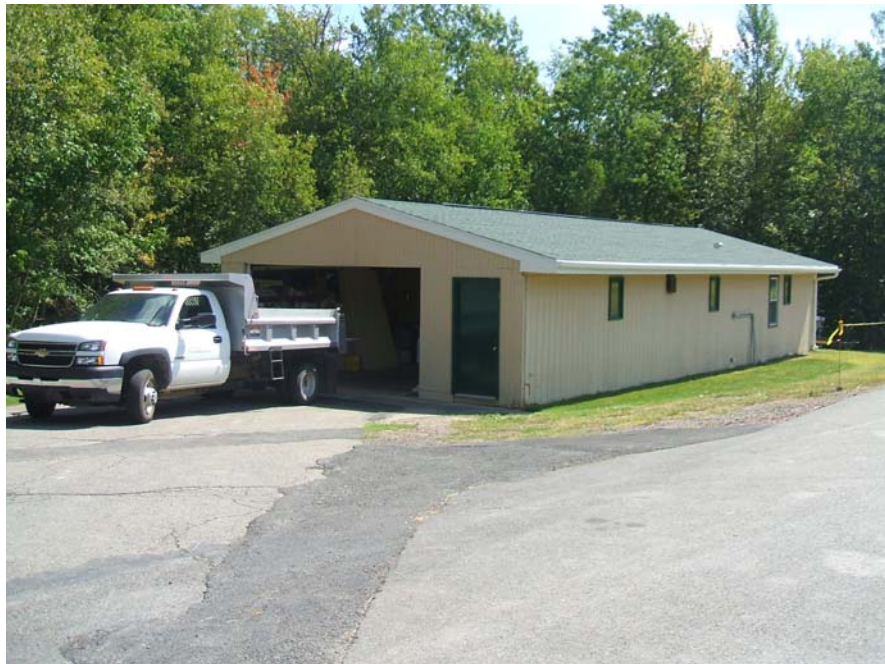
View of Maintenance Building located next to Park Office
