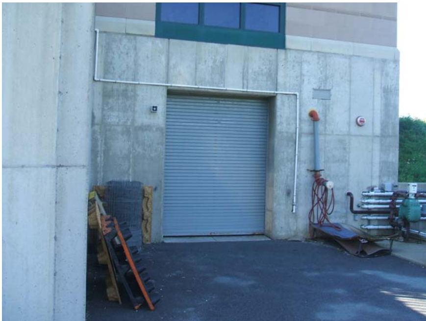
View of loading area with overhead door
