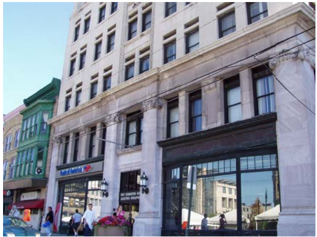
SCRANTON ELECTRIC BUILDING
