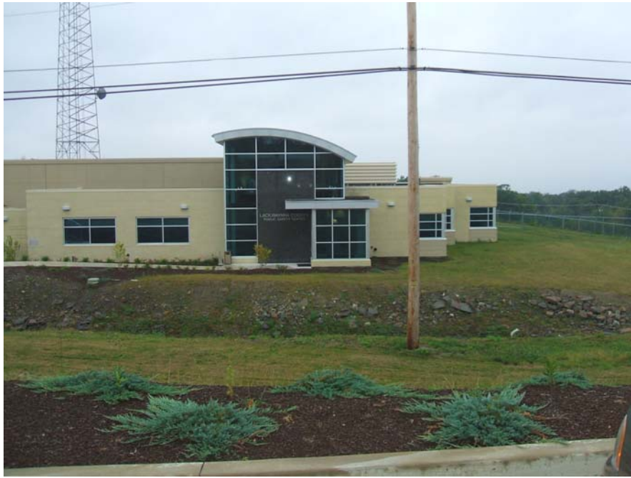
View of building looking southwest, taken from visitors parking area
