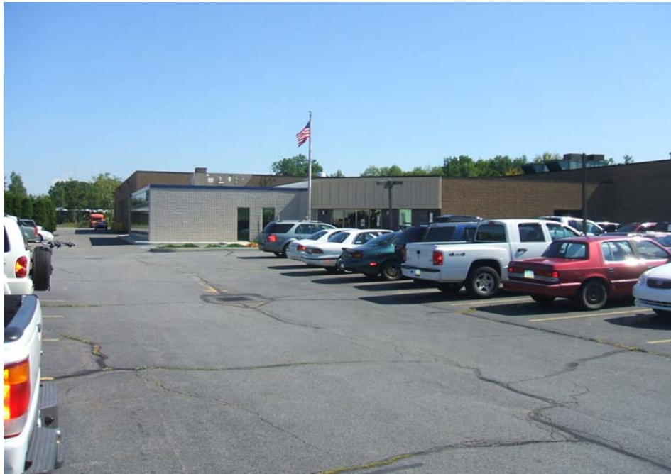
Front view of building taken from parking lot
