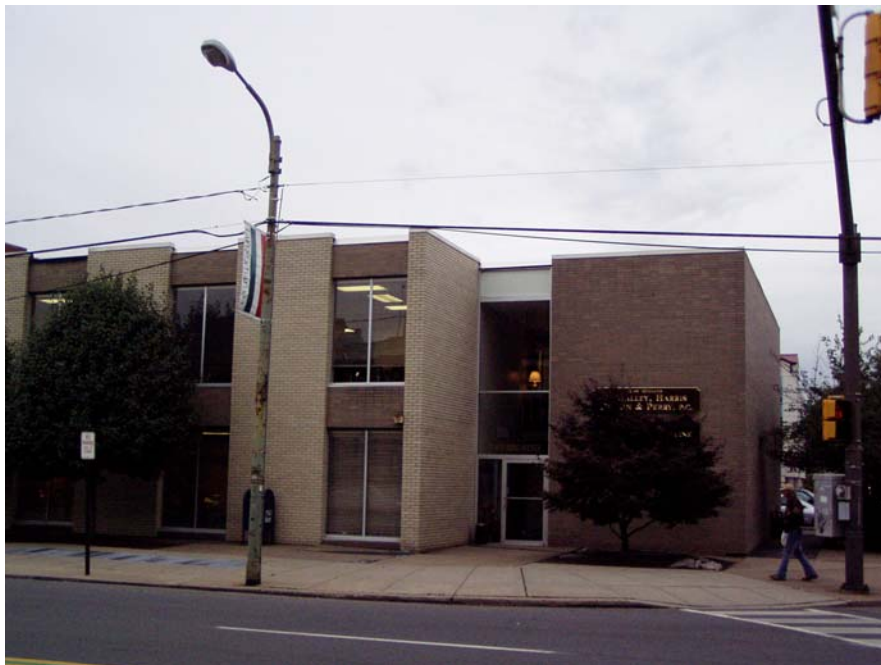
View of front of building taken from across Wyoming Avenue
