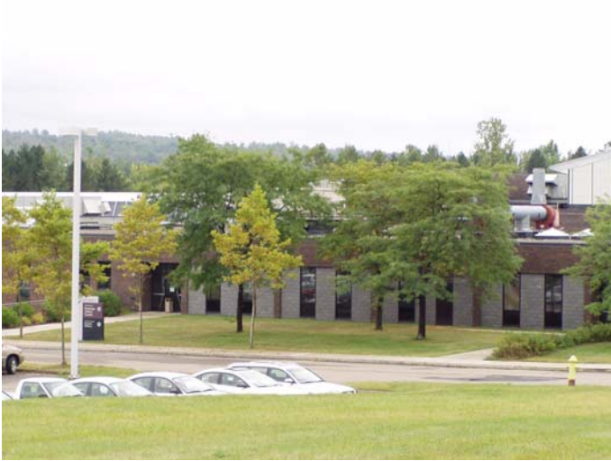
North side of building
