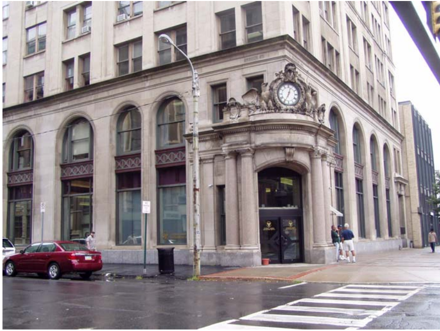
View of building from intersection of Spruce Street and Wyoming Avenue
