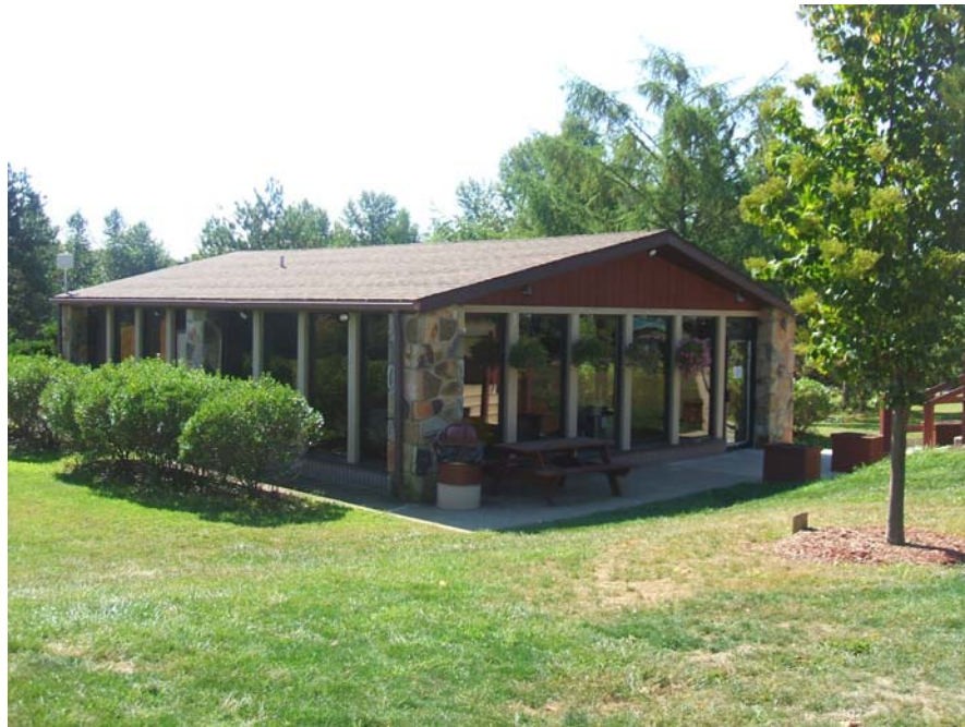
View of Park Office looking southwest
