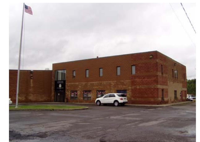
901 ENTERPRISE DRIVE ROADS & BRIDGES
