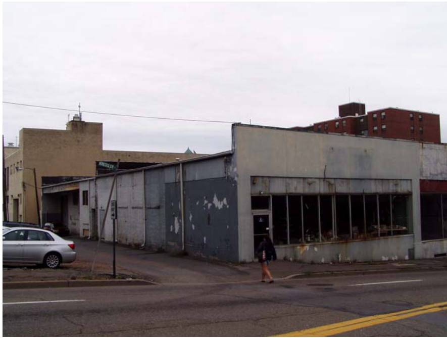
View of side of building from Mulberry Street
