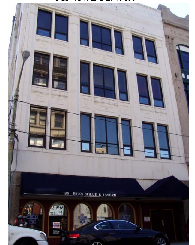
BRIXX BUILDING OCTOBER, 2008
