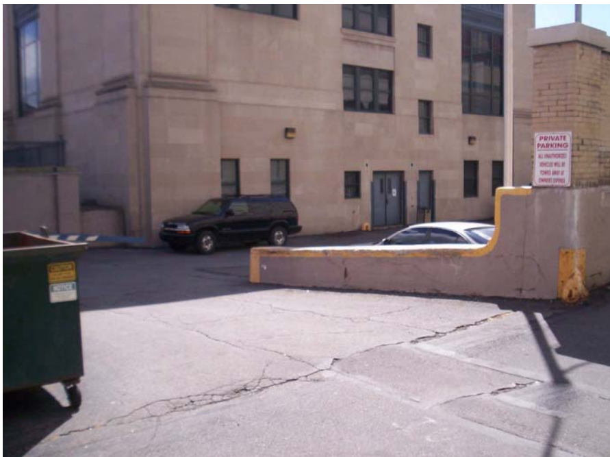
View of rear of building showing parking and loading area
