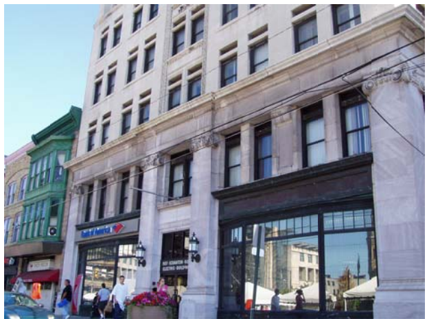
SCRANTON ELECTRIC BUILDING OCTOBER, 2008
