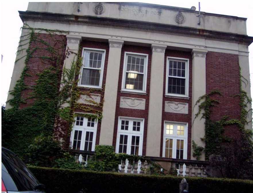
View of front of building from North Washington Avenue
