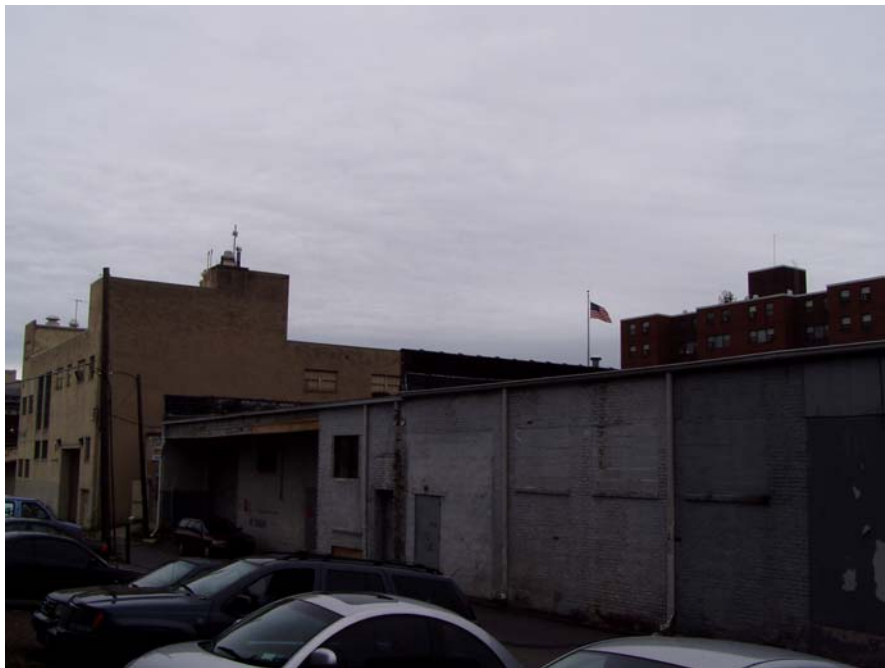
View of back of building from Kressler Court(alley)
