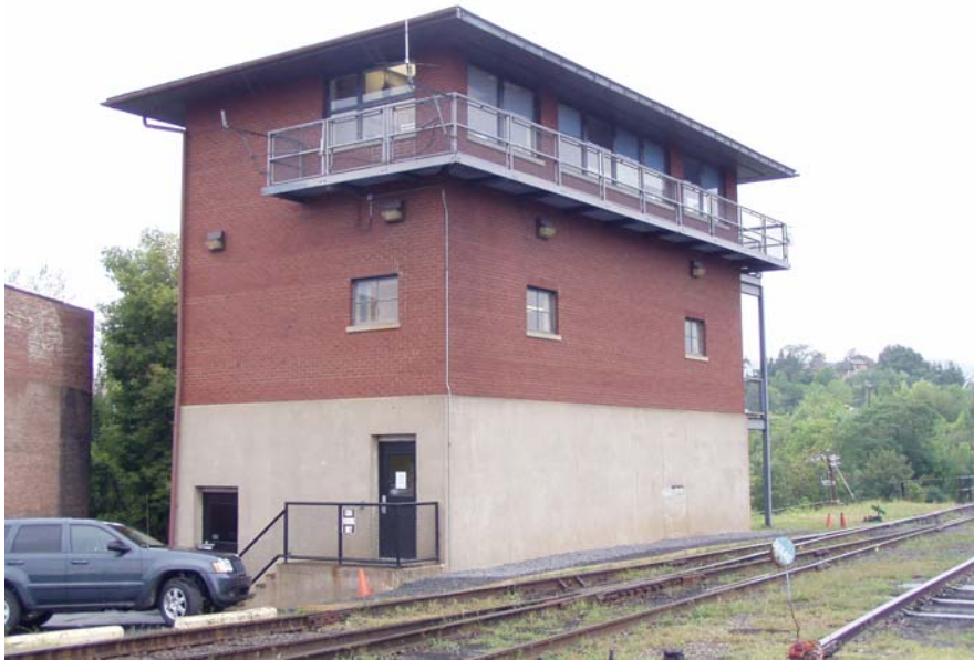
View of Tower facing southwest
