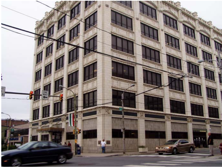
View of building from intersection of Spruce and Adams Ave.
