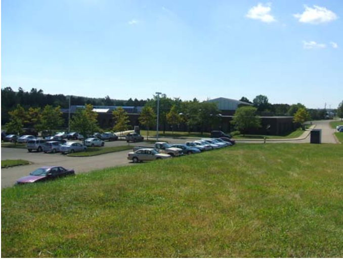
View of building looking south
