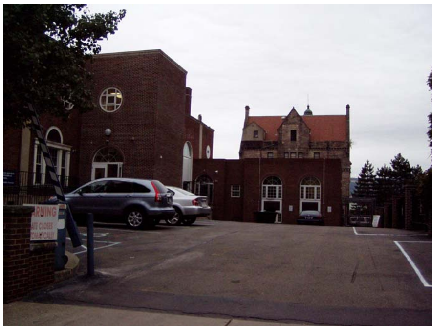
View of parking adjacent to building
