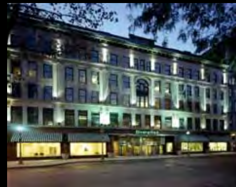
The Globe Store Restoration
