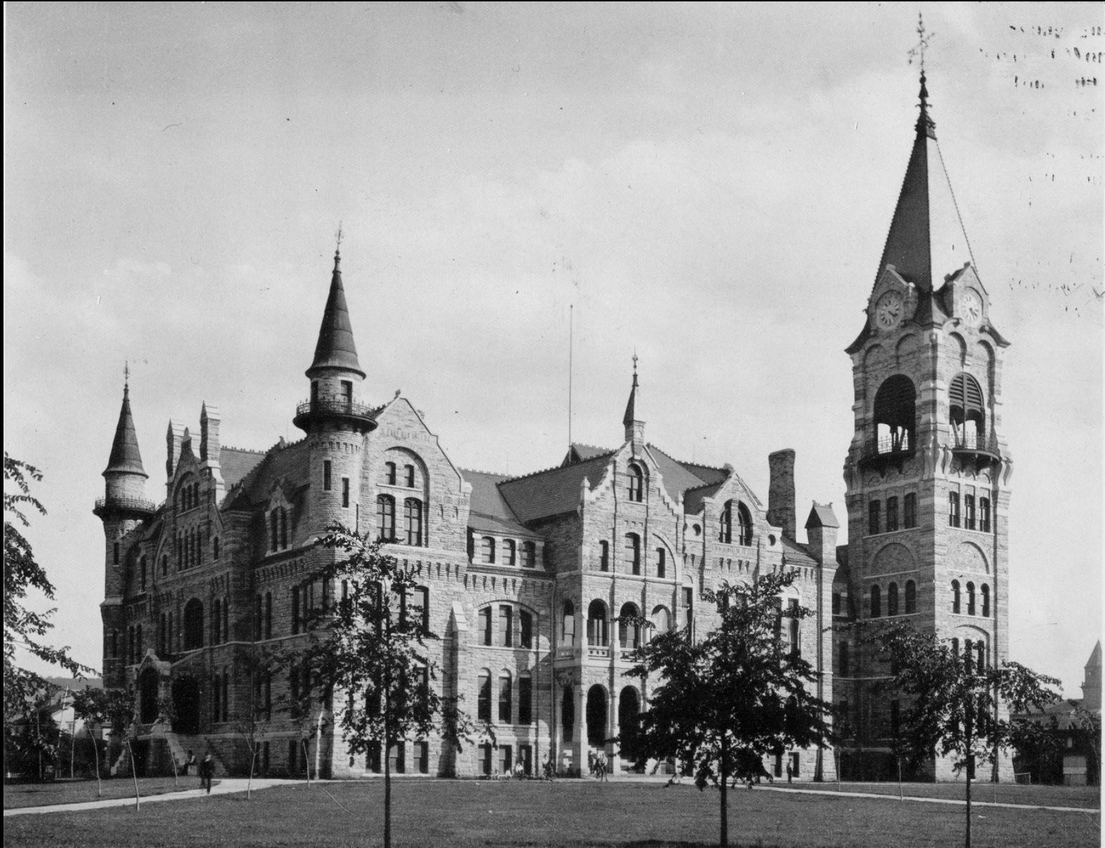
View from North Washington Avenue
