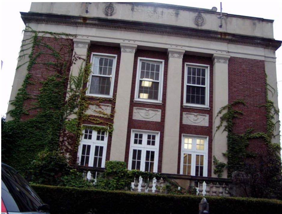
View of front of building from North Washington Ave.
