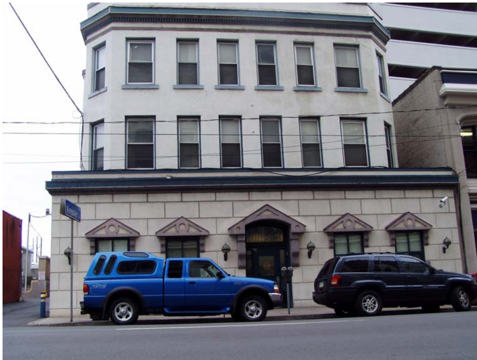
View of front of building from Spruce St.
