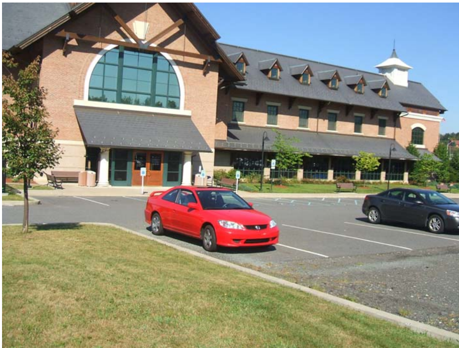
View of entrance looking West
