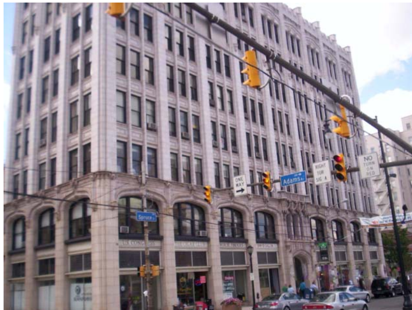
View of building looking along Spruce St
