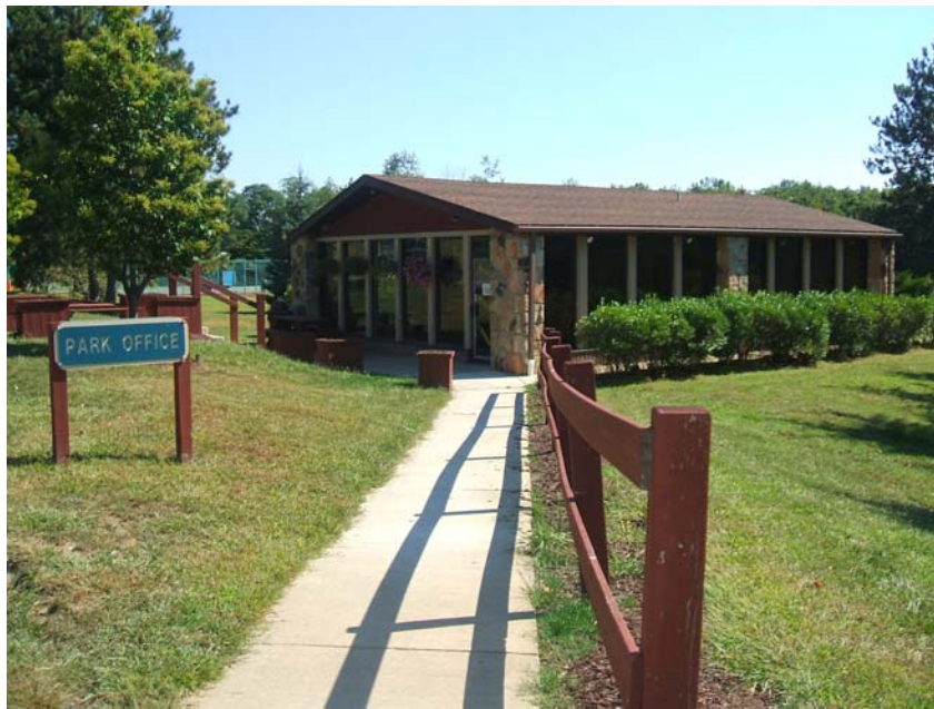
View looking NW showing handicap access to building
