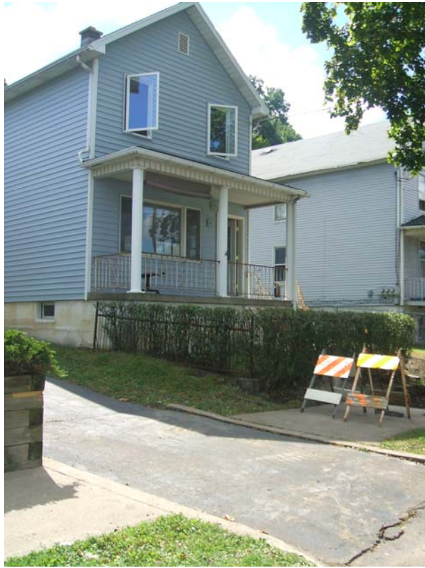
View of building from Wyoming Avenue looking SW
