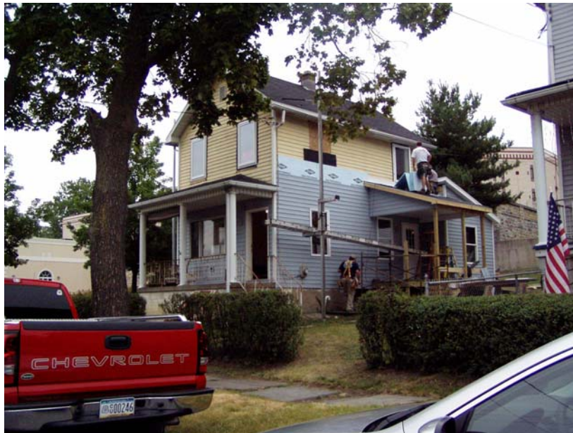
View of building from Wyoming Avenue looking NE
