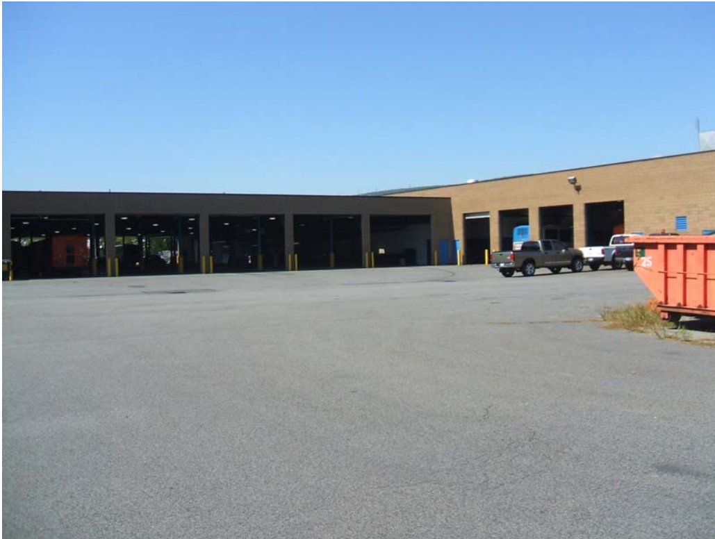
View of garage and repair bays.
