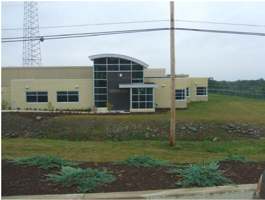
View of building looking SW taken from visitors parking area
