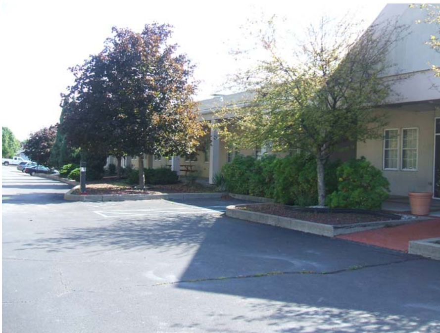
View of building looking NE
