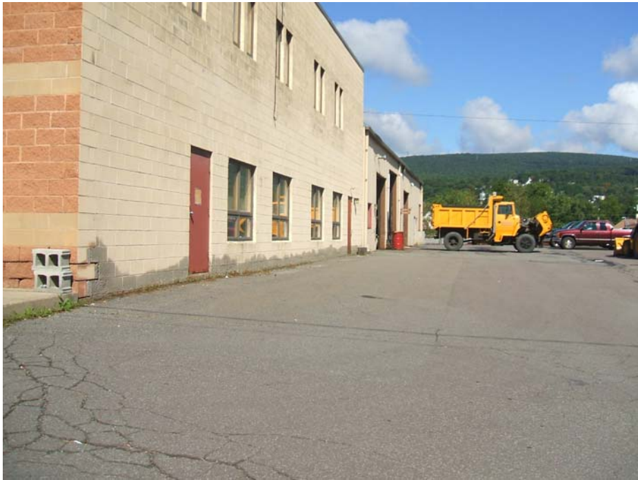
View of rear of building showing loading areas and garage door access
