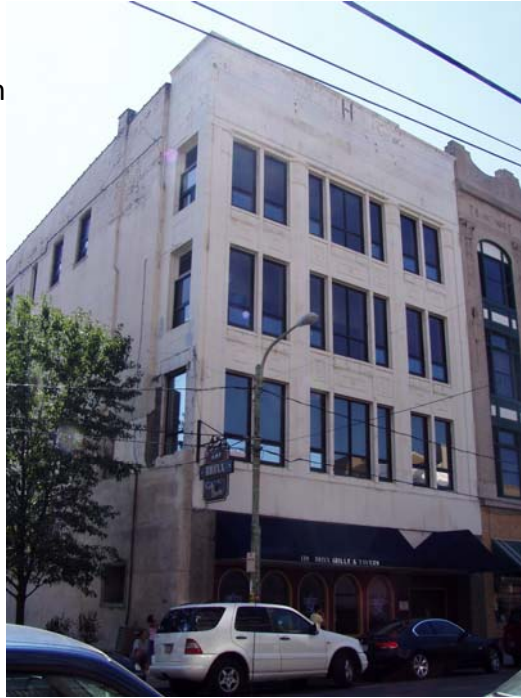
View of building from North
