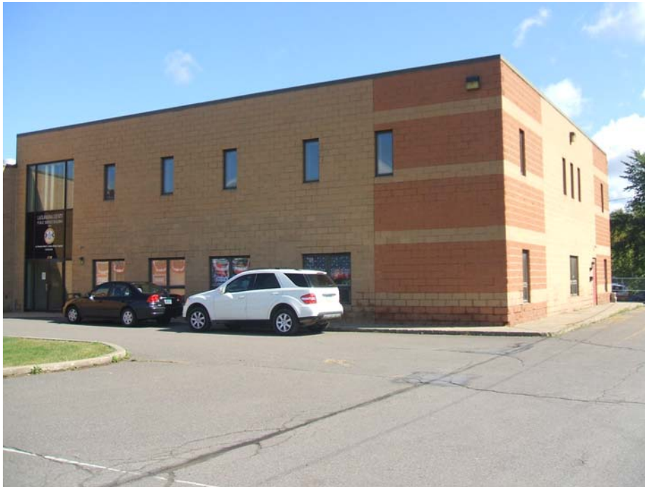
View of front of building from entrance driveway
