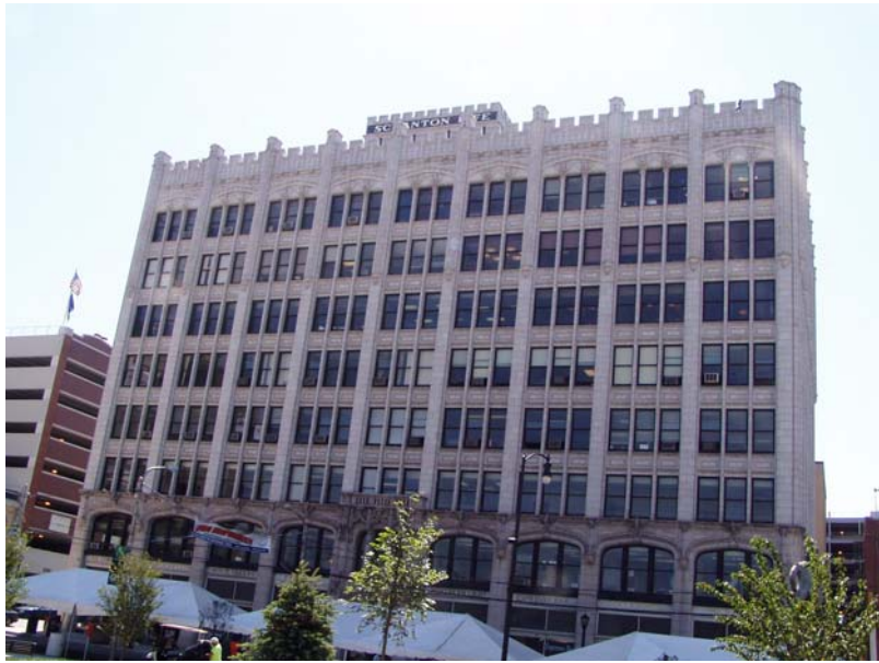
View of building looking across Spruce St
