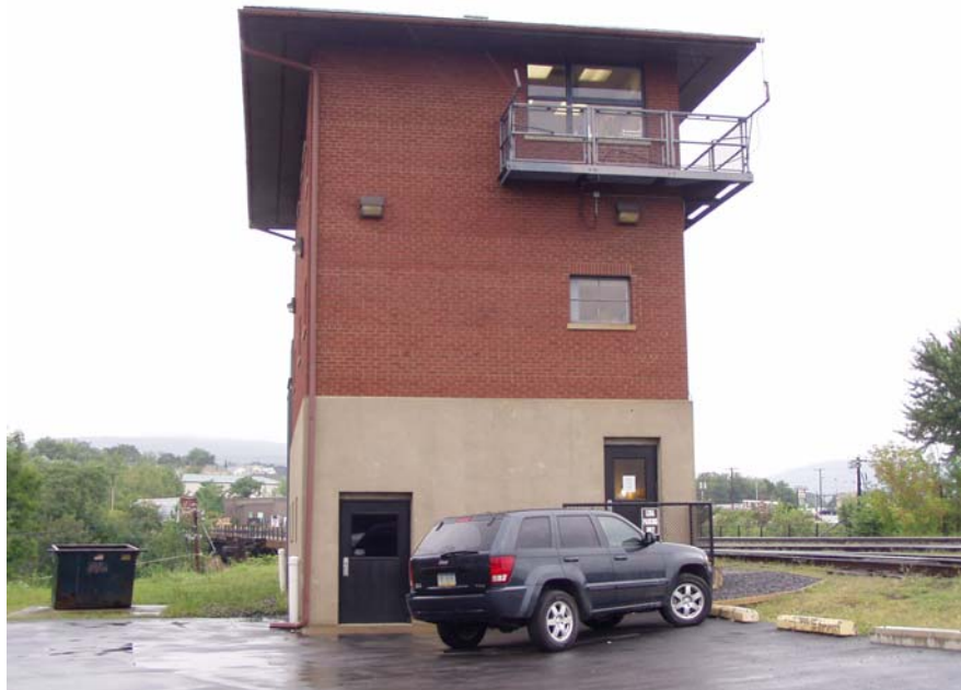
View of Tower facing W
