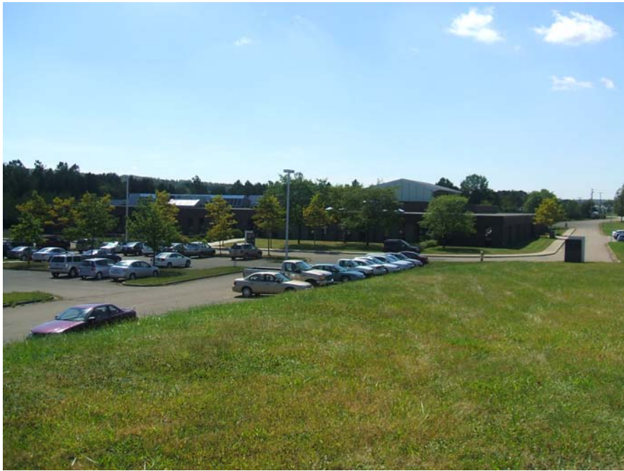
View of building looking south
