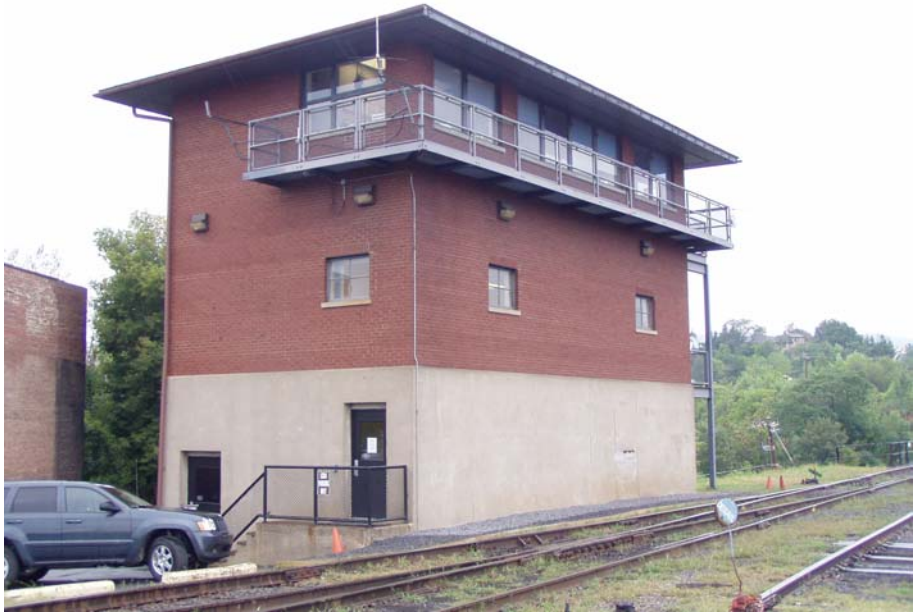
View of Tower facing SW
