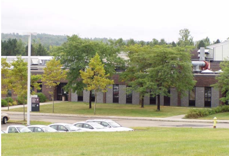
View of the north side of building
