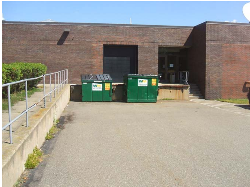
View of building looking north showing loading dock
