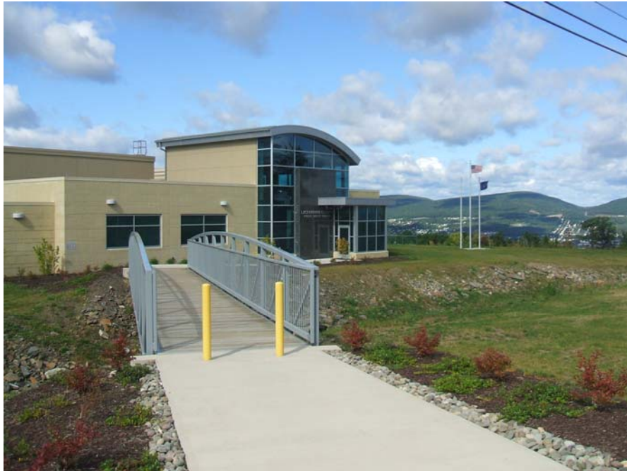
View of entrance showing bridge and handicap access
