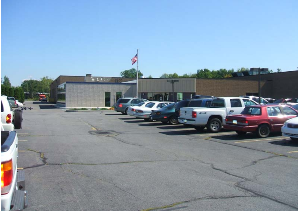
Front view of building from taken from parking lot.
